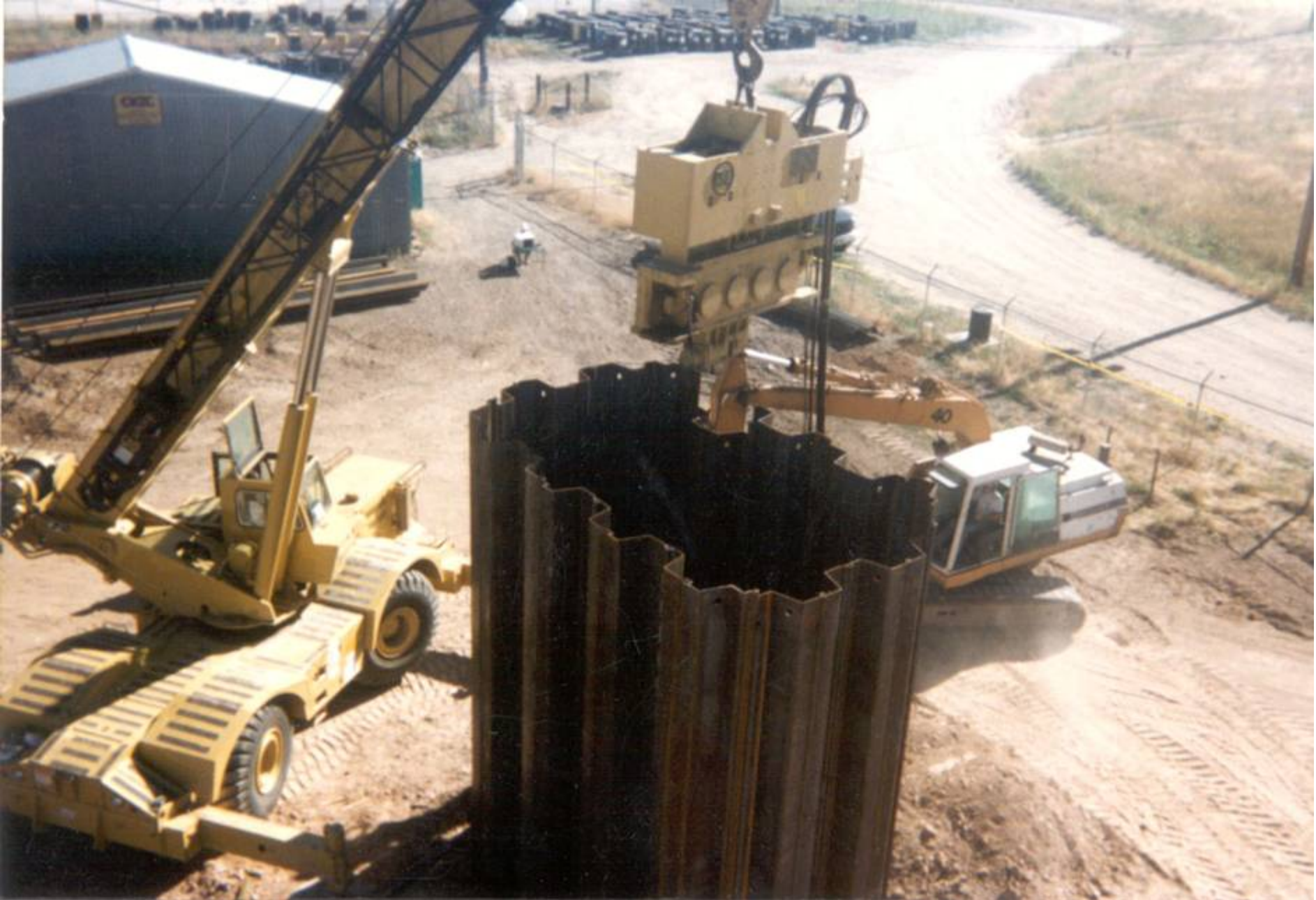
Sheet piles for Air Force missile silos
