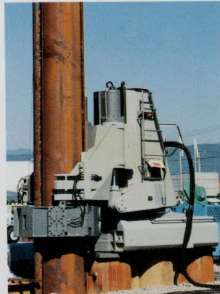
Silent Piler for Steel Tubular Piles Only
