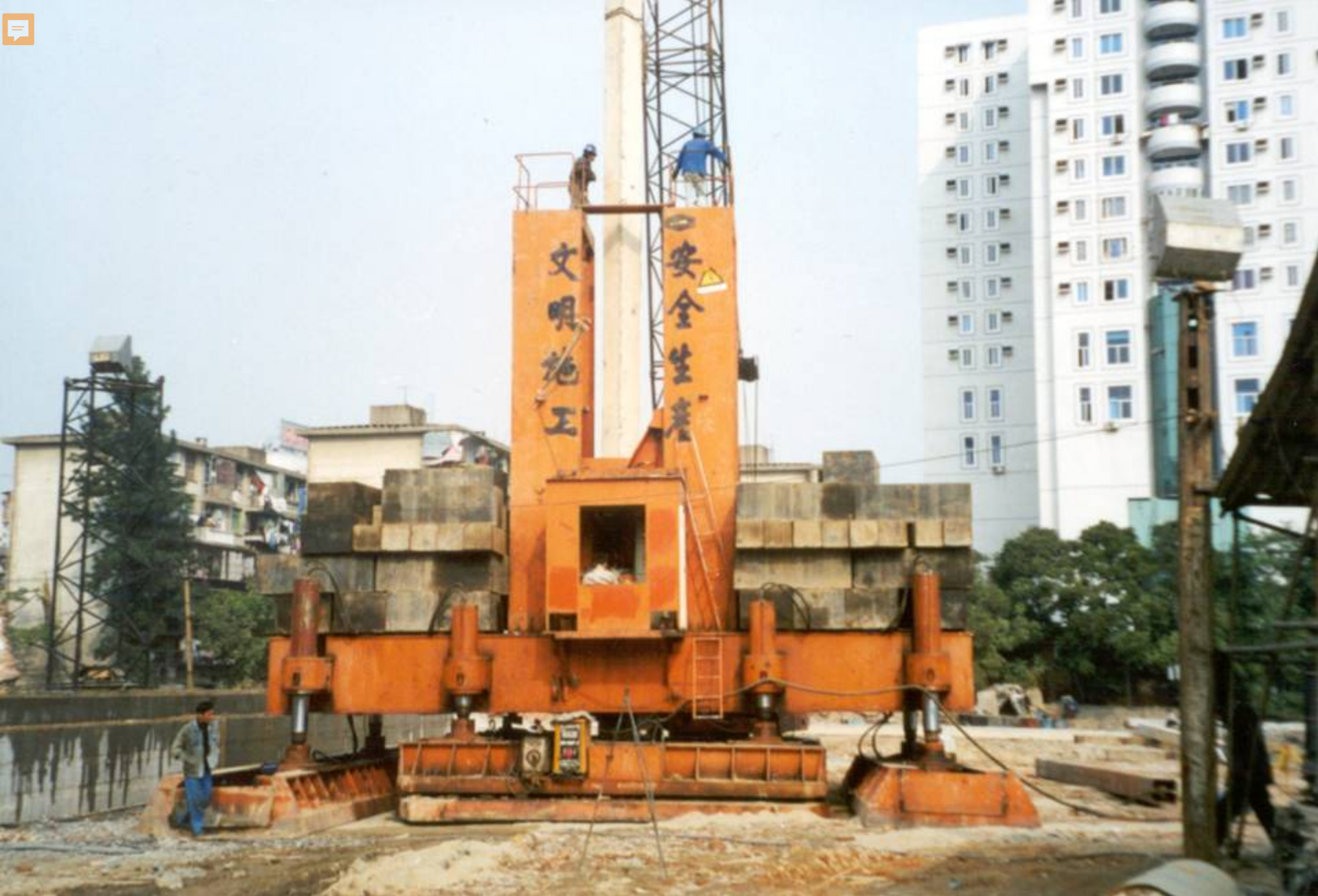
21 inch square pile being pressed into the ground
