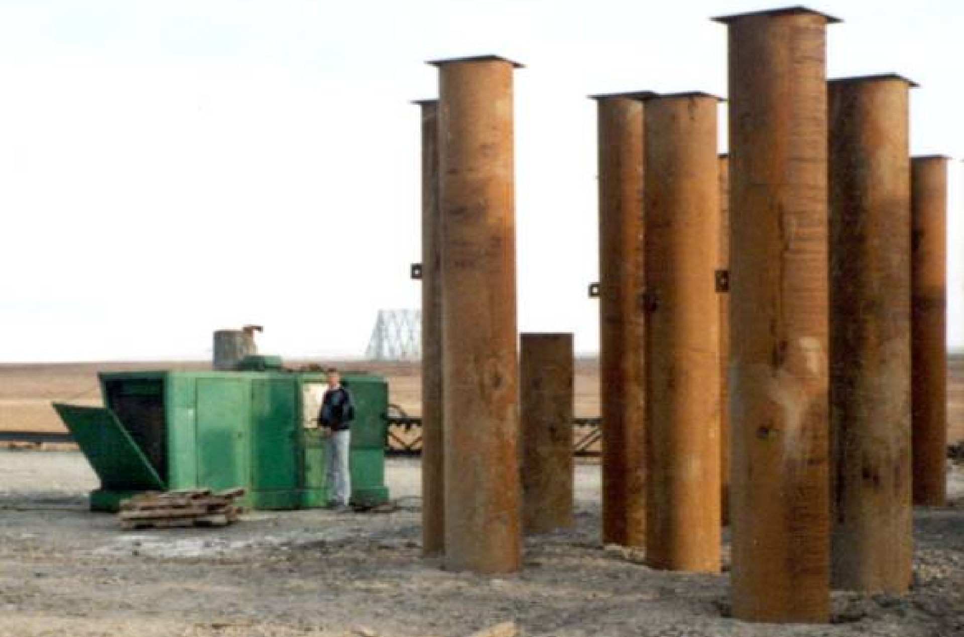
Large diameter pile piles for a bridge in Vancouver, B.C.
